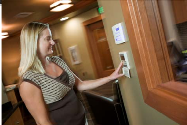
The entire Daikin system, which stands completely alone from the rest of the building's MEP systems, is controlled via Daikin remote sensors and 7-day programmable controllers.
