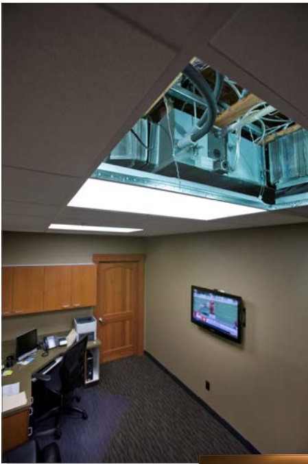
The entire Daikin system, which stands completely alone from the rest of the building's MEP systems, is controlled via Daikin remote sensors and 7-day programmable controllers.
