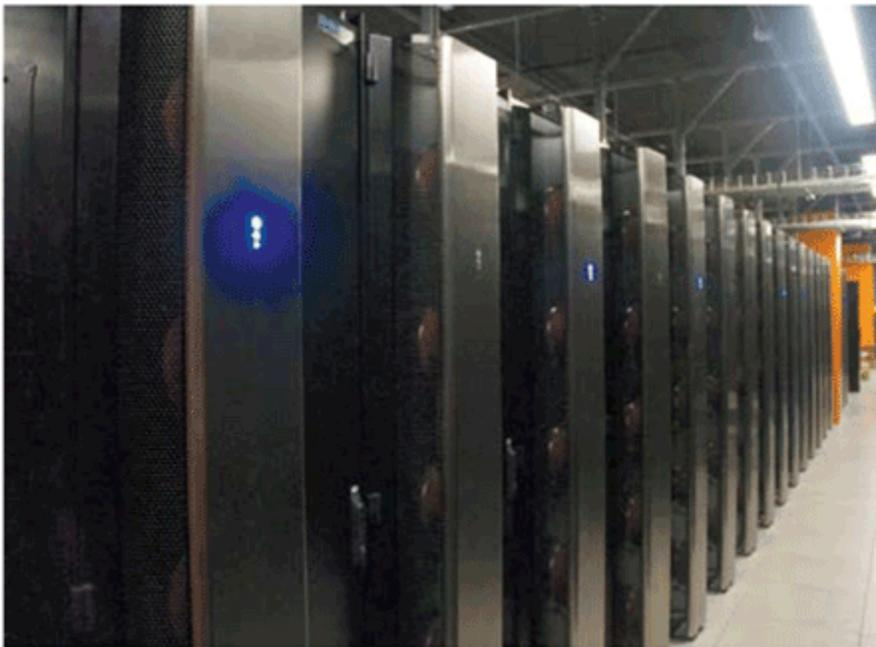
**Chilled Door high-density rack-cooling units.**
